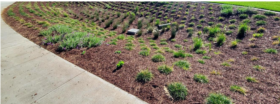
Example of stormwater basin.
